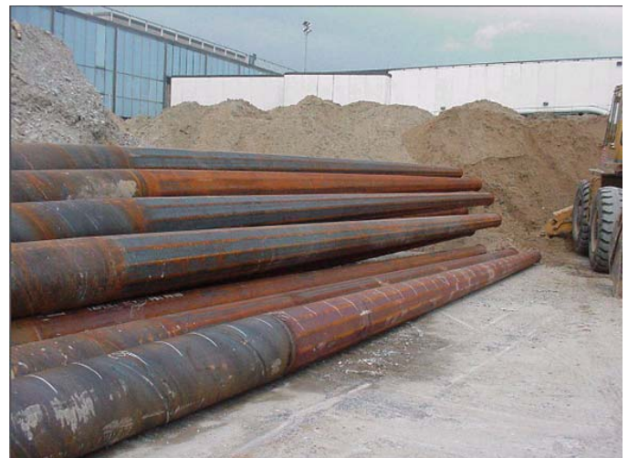
Fig. 2. Type II Tapertube Piles Stockpiled at Job Site and Ready for Installation.
