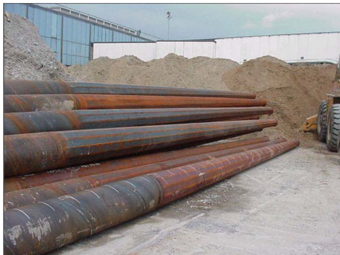
FIG. 1. Tapertube TM Piles Stockpiled at Job Site and Ready for Installation
