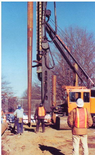
FIG 4. Tapertube Pile Being Positioned for Driving
