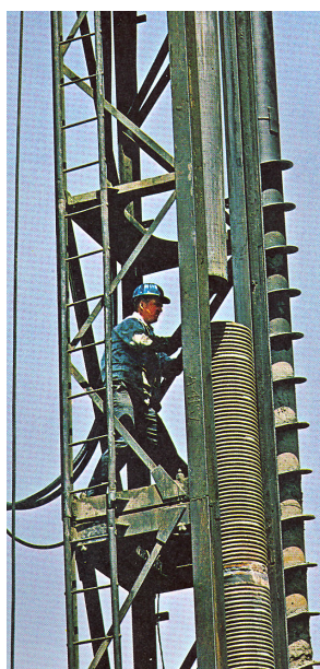
FIG. 2. Raymond Step-Taper Pile Being Readied for Installation
