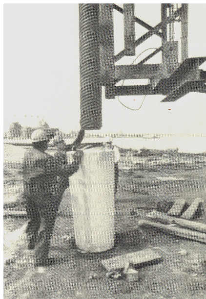
FIG. 5. An Early Version of a TPT Pile Being Assembled Prior to Driving
