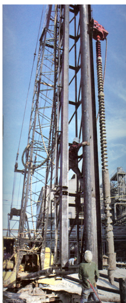
FIG. 1. Creosote-Treated Timber Pile Being Readied for Installation
