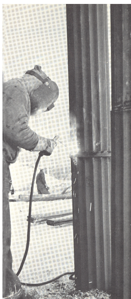
FIG. 3. Partially-Driven Monotube Pile Having a Constant-Diameter Upper Section (Extension) Being Field Welded to the Tapered Lower Section
